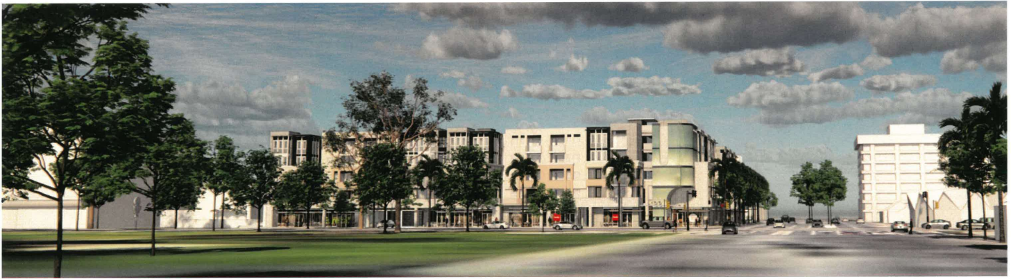
3. VIEW FROM ARCADIA STATE PARK
