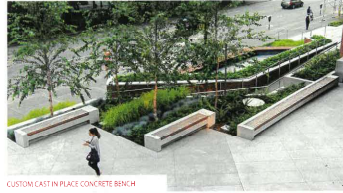
CUSTOM CAST IN PLACE CONCRETE BENCH
